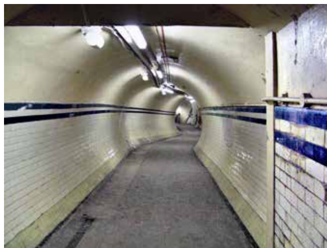
The winding passage leading from the lower lift landing to the stairs down to Platform 1. Nothing has changed here since closure in 1994. Photo James Buller
